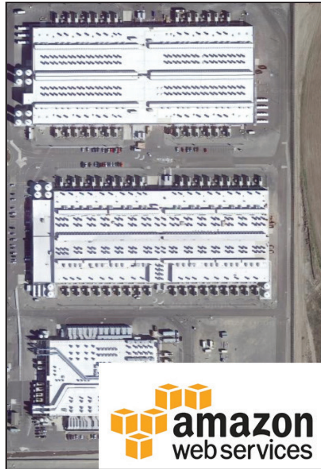
Pictured are a couple of the large Amazon Web Services data centers at Boardman.
