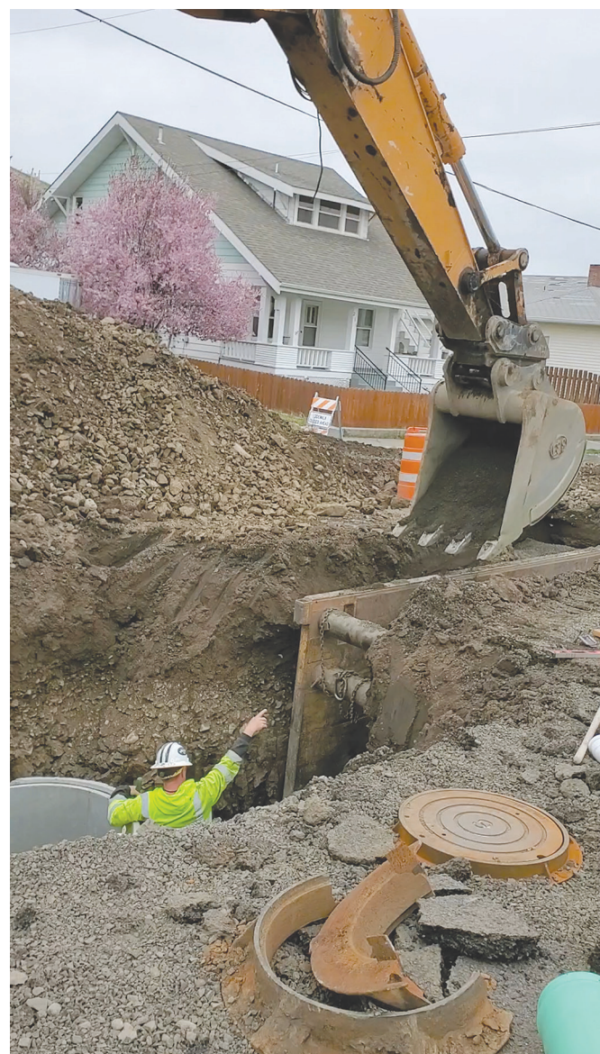
Workmen dig deep to replace sewer lines at the corner of Gale and Willow Streets. They are hitting more rock than originally anticipated.
