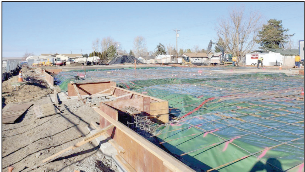
Construction has started on the new county office buildings in Irrigon.
