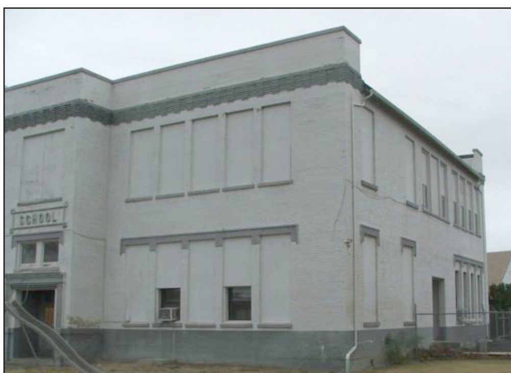
If local businessman Sam Bellamy's plans work out, this old Lexington School building will have new life as a short-term visitor business.
