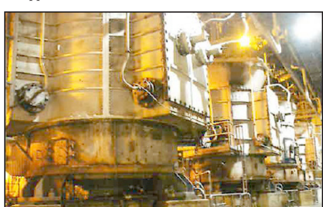
All the equipment in the plant will be decommissioned and either scrapped or demolished.
