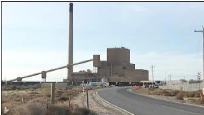
The PGE coal plant in Boardman prepares for closing.
