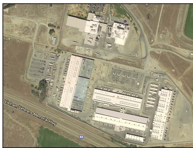
Aerial shot of a typical Amazon data center built on Hwy 84 near Boardman.
