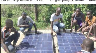
Getting ready to install the solar panels that will power pumps to replace hand pumping
