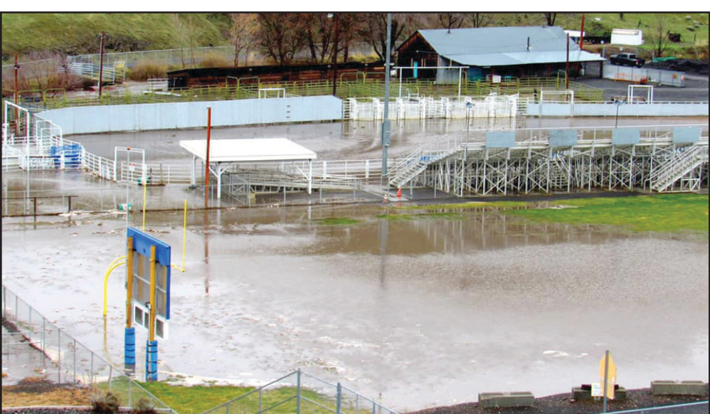
The arena at Morrow County Fairgrounds and Les Payne field suffered some damage when Hinton Creek flooded it recently. According to Darrell Green county administrator some water made its way inside the fair office, but they will be waiting until the water subsides to assess any damage. Electricity was shut down for a short time due to a power pole being flooded and the RV park sustained a little damage.
