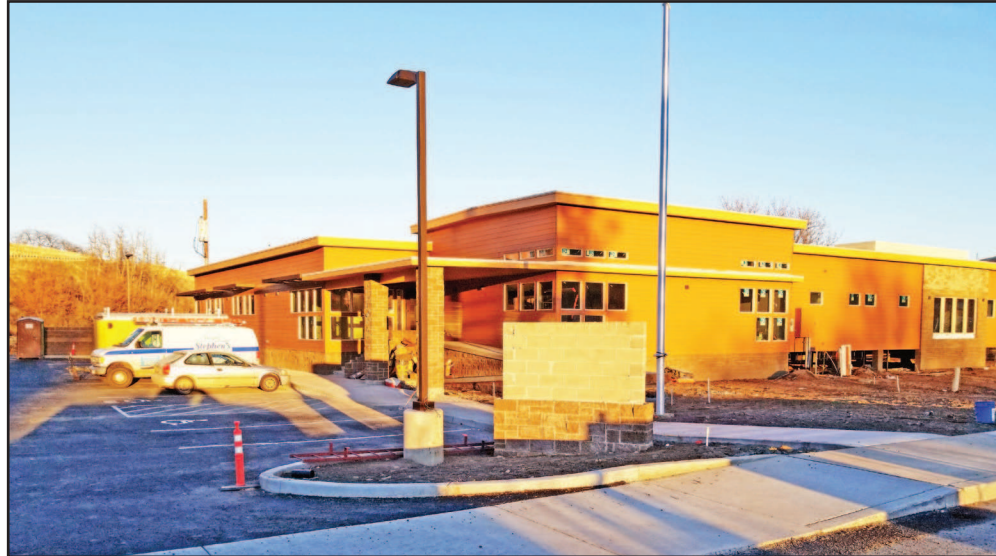
Community Counseling Solutions new offices on Sperry Street are nearing completion. CCS plans on moving here in June. -Photo by David Sykes
