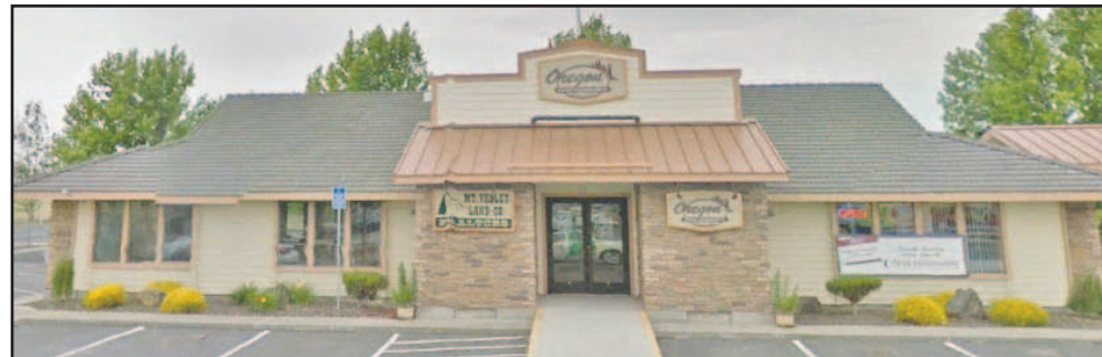
Morrow County Health District is in the process of remodeling the former Mountain Valley Land Company building. -Contributed photo
