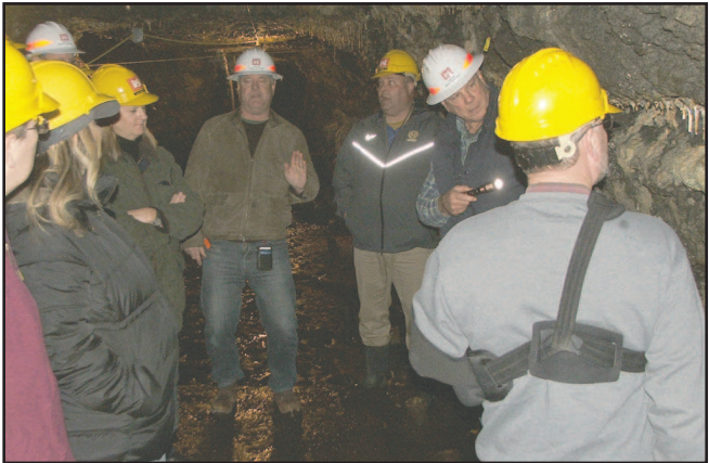
Inside the tunnels which run the length of the base of the dam. -Photo by David Sykes
