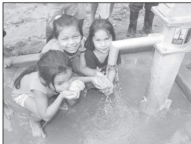
A group of young girls in Sol Naciente, Peru, enjoy water from the new pump installed through the work of Living Water International and Heppner's Shared Ministry. -Contributed photo
