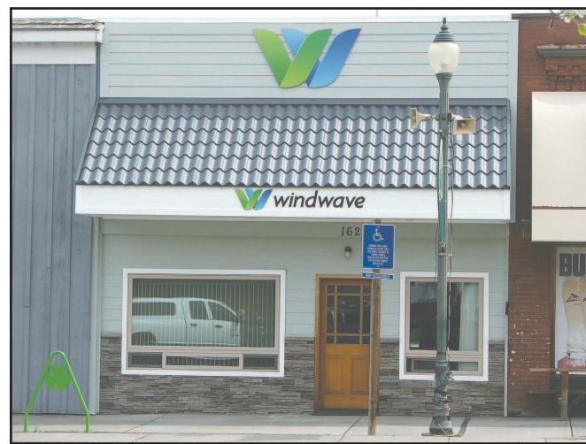
Morrow County Health District has purchased the Windwave building on Main Street in Heppner for use in the district's home health and hospice program. -Photo by David Sykes
