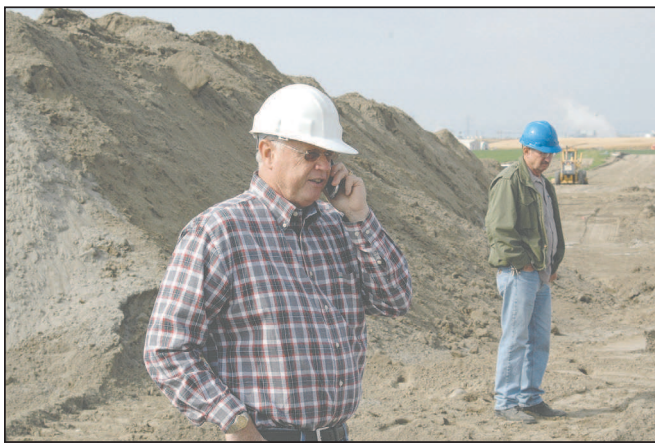
Port of Morrow General Manager Gary Neal checks out a construction project at the Port. The Port is working in collaboration with local educators to better train local youth in preparation for the new jobs becoming available there. -Contributed photo
