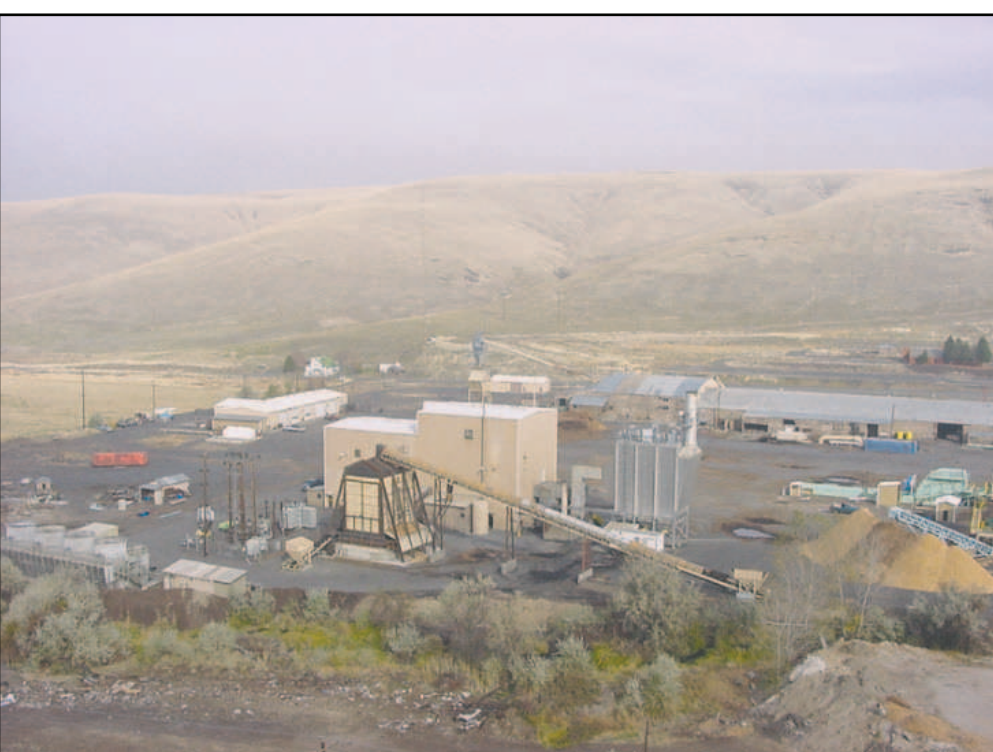
Precision Energy Services of Hayden Lake, ID is looking into purchasing and starting up the long dormant wood-fueled power plant at the former Kinzua Mill site in Heppner.
