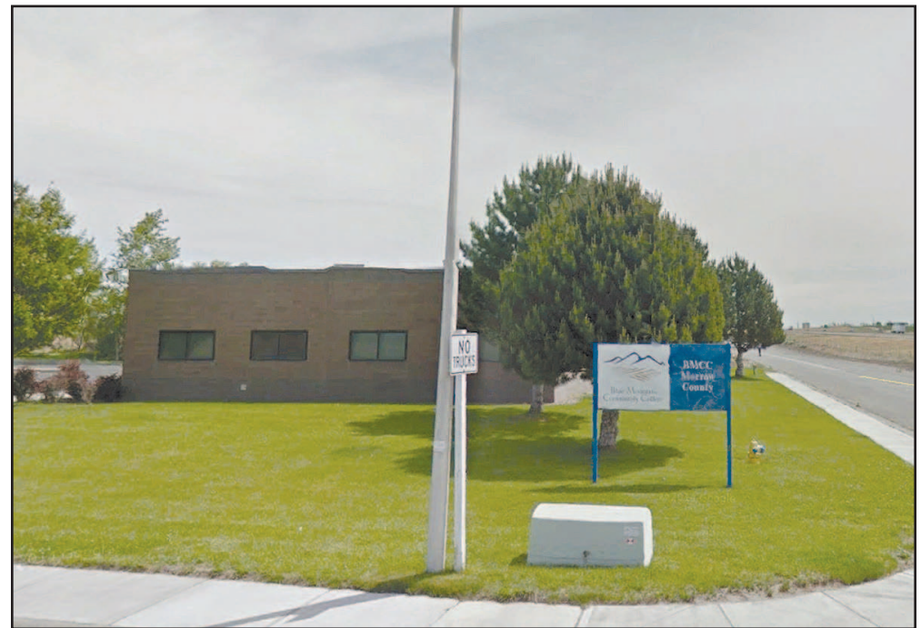
The county is considering purchasing BMCC's Boardman facility on Front Street, which becomes available in 2017.
