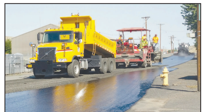
ODOT's chip-sealing project on Heppner's Main Street got into full swing Monday. -Photo by Megan Futter
