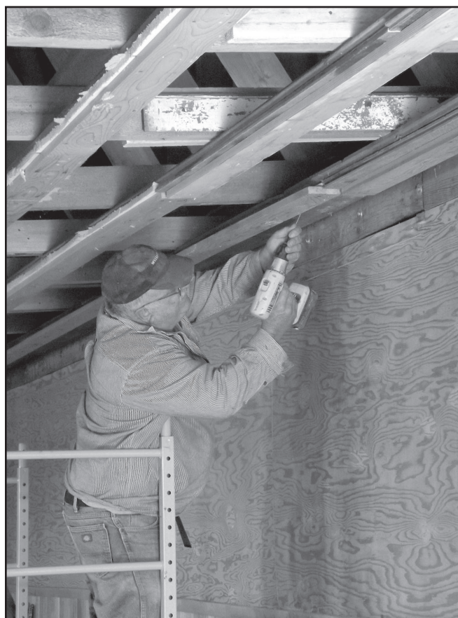
Rick McDaniel working at the Hardman Community Center. -Contributed photo
