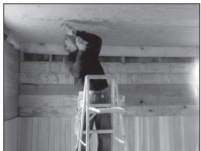
Scott Smythe getting started on the ceiling tear out. —Contributed photo
