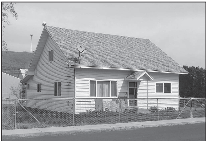
This house in Ione has been purchased for the town's school-based clinic site. -Photo by David Sykes
