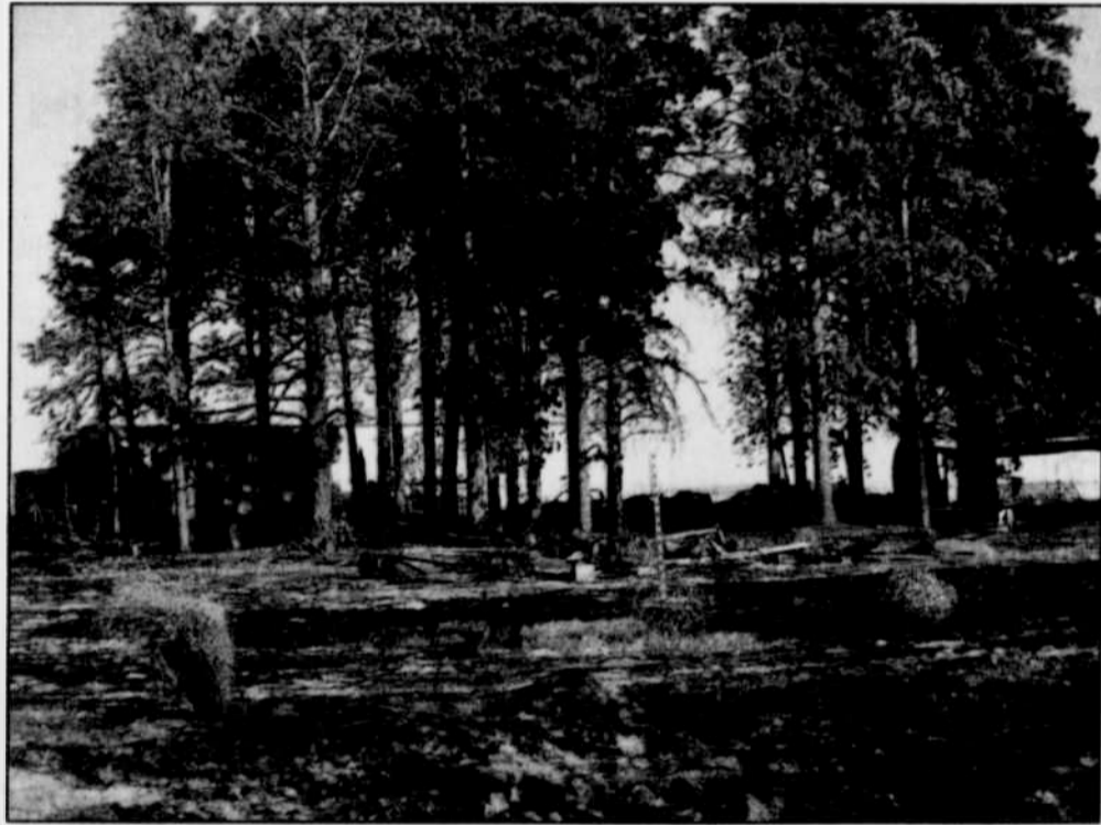
A burned and twisted pile of metal is all that remains in the wake of last week's fire, which came dangerously close to doing even more damage. -Photo by David Sykes
