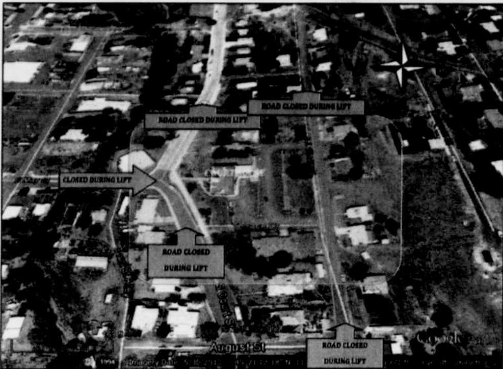
Streets in the area of the courthouse in Heppner will be closed during the lift planned for June 26. -Contributed photo
