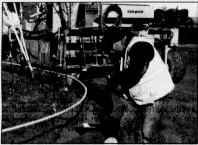
Workers pour concrete for new curbs, gutters and sidewalks on Riverside Street in Heppner. The work is part of the larger street and sidewalk renovation project now going on along Riverside and Water streets. Van Nevel Concrete and Curbing of Terrebonne, Ore. is doing this curbing work using a large machine (see above) being fed wet concrete by a mixer truck. -Photo by David Sykes
