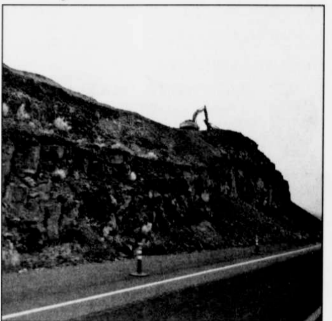
Backhoes like this one have become a familiar sight near milepost 35 on Hwy. 74, where travelers between Lexington and Ione can expect short delays, usually between 10 and 15 minutes. The work is part of a rock-fall project that will cut back part of the rock face to help reduce the amount of falling debris onto the highway. Work is expected to be complete by mid-march. -Photo by April Sykes
