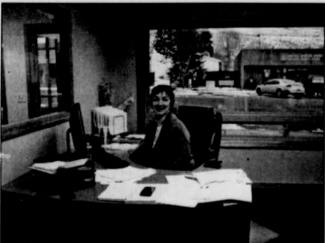
WindWave employees demolished their offices during the first part of November, in preparation for a remodeling project. A carpenter began work November 8. The staff moved back into the building on December 16. Bottom Photo: Pat Lauritsen, general manager - Photos by Autumn Morgan
