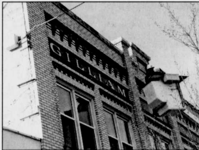
With the help of Columbia Basin Electric and Rod Wilson, members of the Farm Foundation replaced the dilapidated sign on the front of the Gilliam Building in Heppner on Friday, March 5. Bob Harrison and Butch Laughlin put together the new gilded letters for the new sign going up on the national historic building. -Photo by David Sykes
