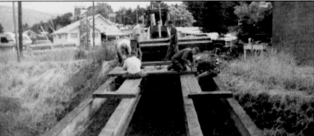
July 4, 2007 - Kirk Street Bridge was in bad need of repairs. Neighbors and the city crew stripped off the old timbers on Sunday and put on a brand new surface on Monday.
