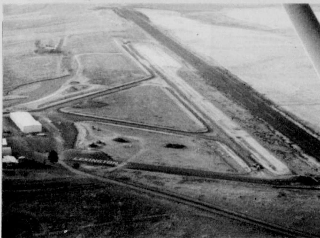
Arial view of Lexington Airport improvements. New taxiway (center) was moved away from main runway (right) and reconstructed. Other new taxiways and new hangars (building at left) have also been added.
