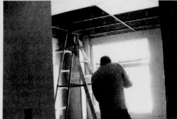
Repairs are underway at the St. Patrick's Senior Center.
