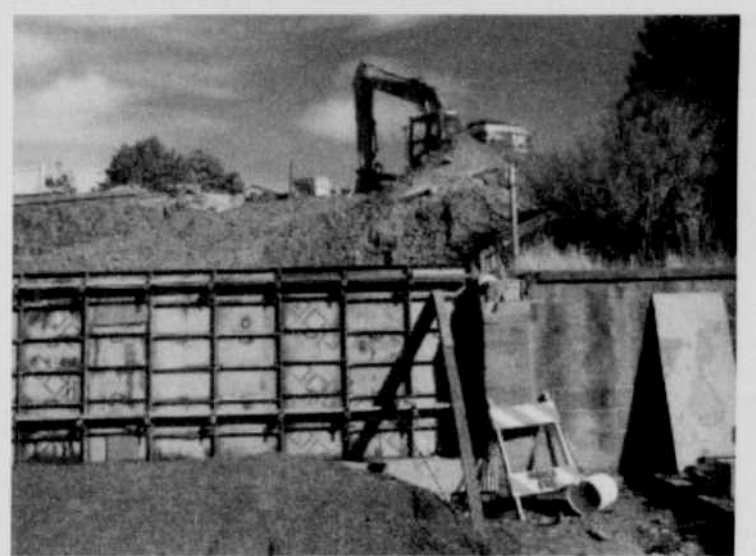
Phase I of Morrow County Courthouse grounds renovation project
