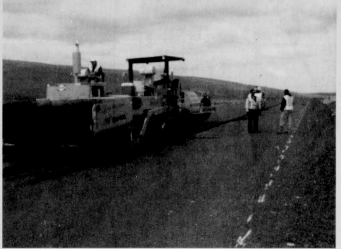
Pavers work at laying asphalt at the new Heppner High School track.
