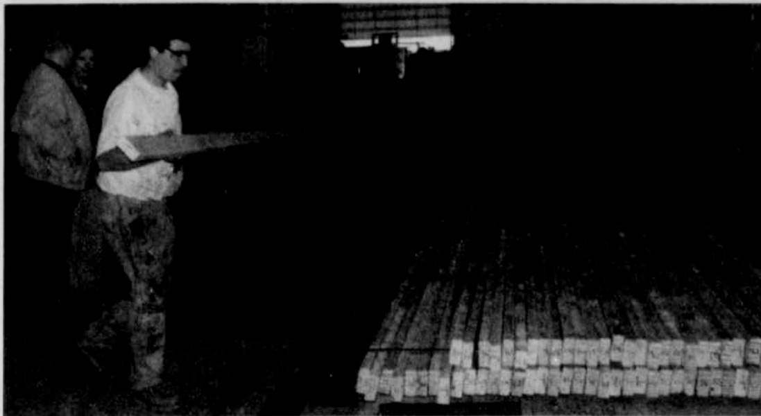
Worker pulls 60-ft 2x4 after lamination
