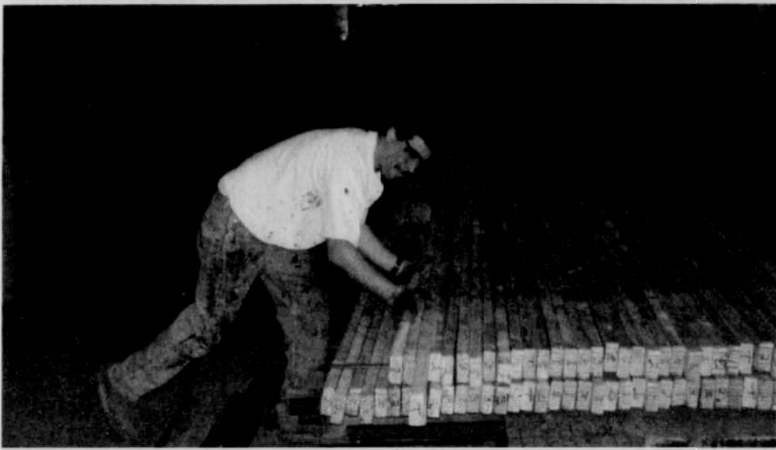
60-ft 2x4s are stacked together in preparation of making larger laminated beam
