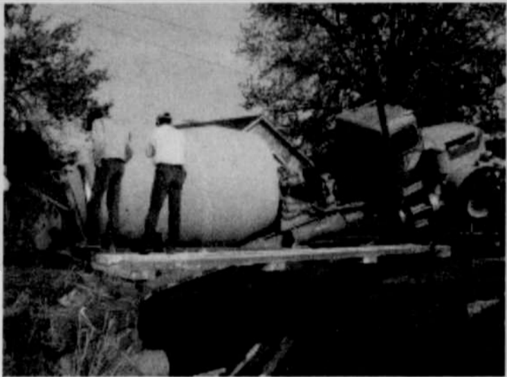
Miller and Sons Excavating use a track hoe to remove a cement truck that went through a wooden bridge in Heppner.
