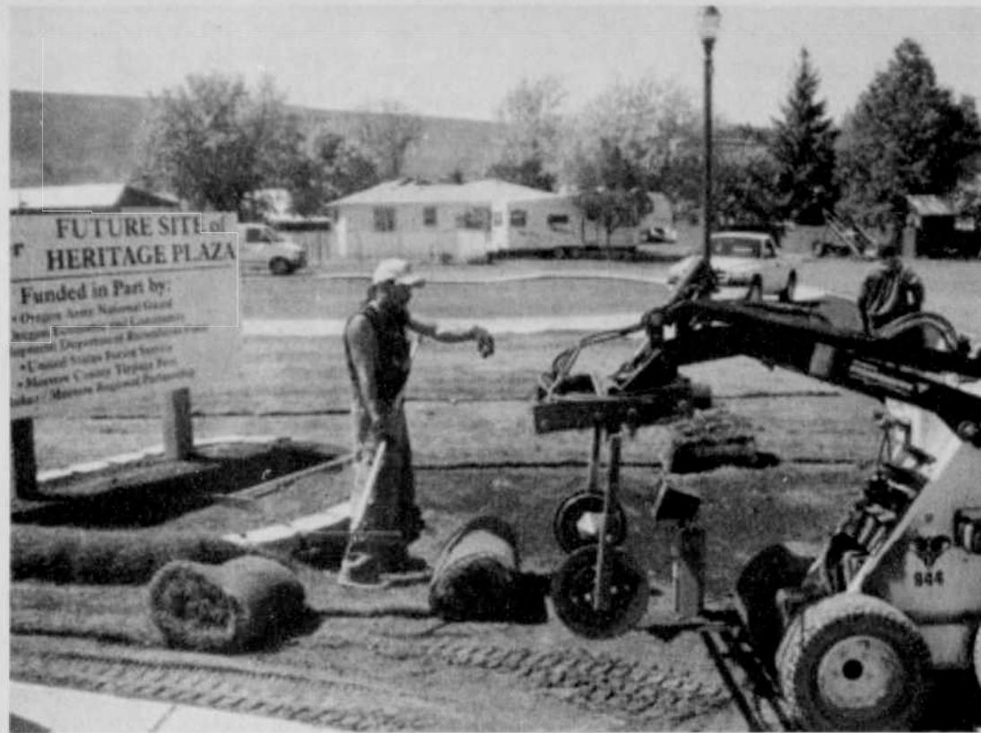
A crew from west Wind Nursery of Hermiston lays sod at Heritage Plaza.
