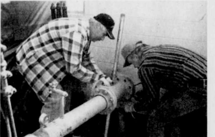
Sam Bellamy (right) and Mark Andrews work on the pump
