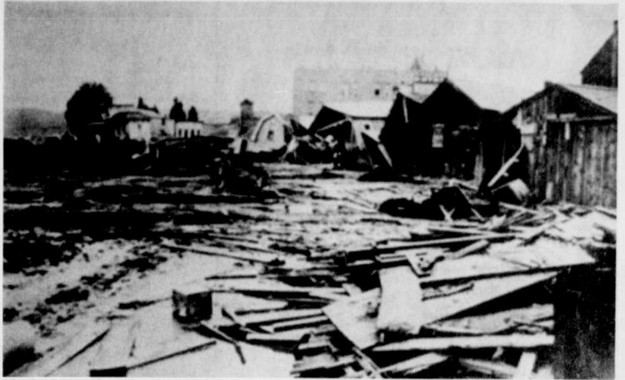
Massive damage from Heppner's 1903 flood
