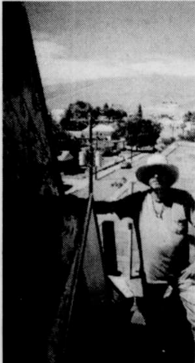
Mark Bruno with new steeple at Heppner Methodist Church
