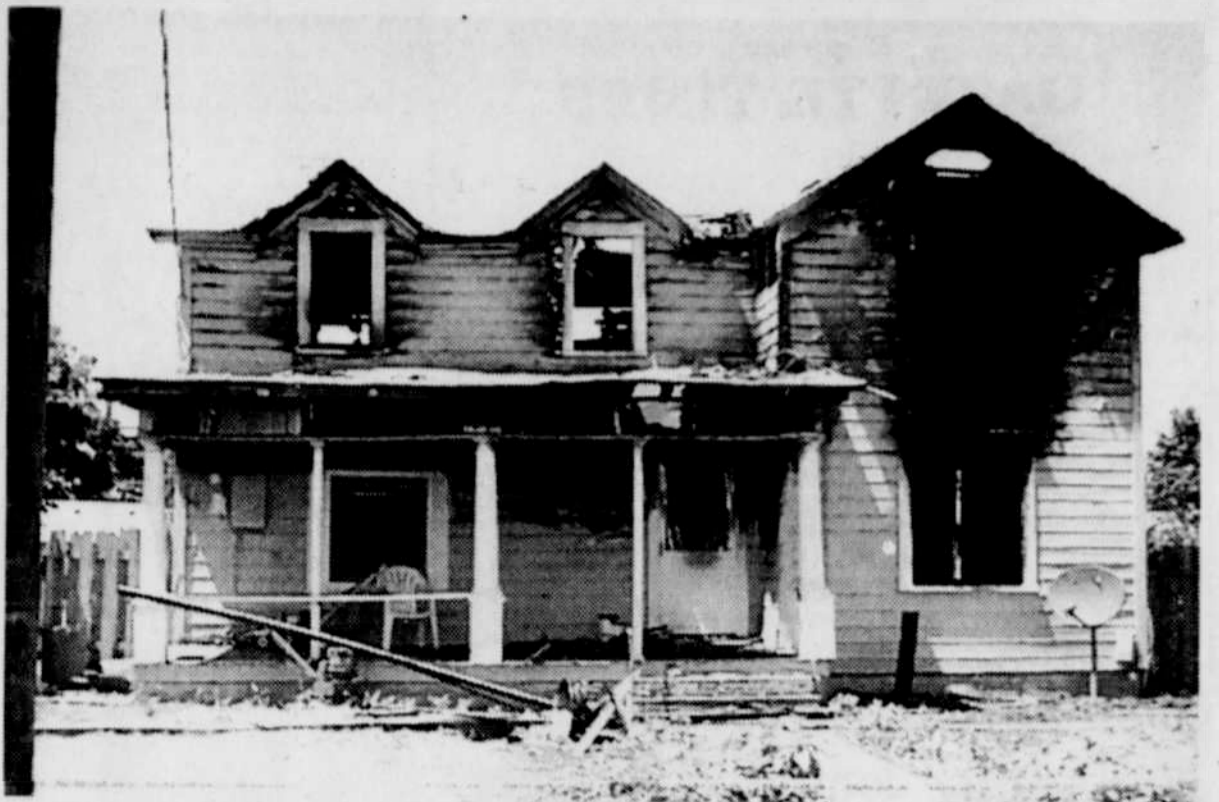
Early morning fire gutted this home on Gale street in Heppner last Friday.
