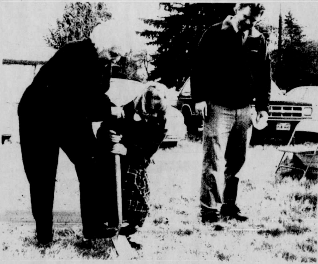
Dot Halvorsen and Brenna Rietmann break ground for the new United Church of Christ building in Ione while the Rev. Paul Clay looks on.
