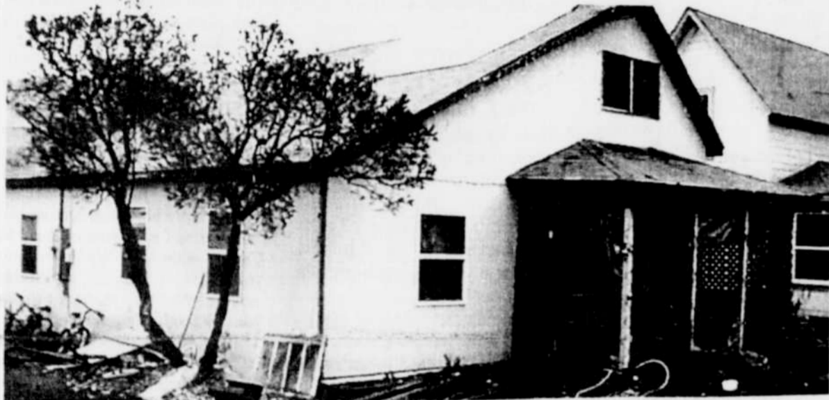
House damaged in fire
