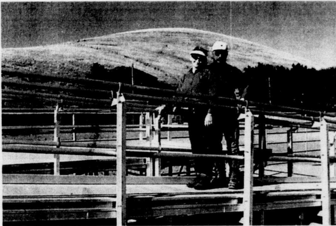
Mary Ann and Barry Munkers show the new handicap ramp and viewing area at the Morrow County Rodeo Grounds. The ramp and viewing facility are just two of the many improvements made by the Rodeo Committee over the past year.
