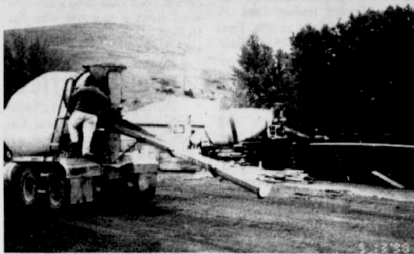
Work continues on the Wilkinson arena
