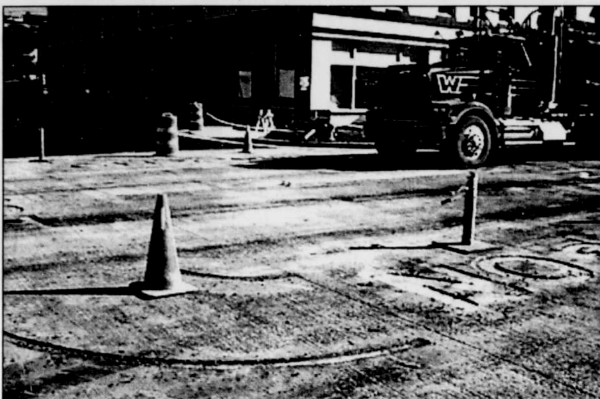
Cement Heppner logo at intersection of Main and Willow streets.
