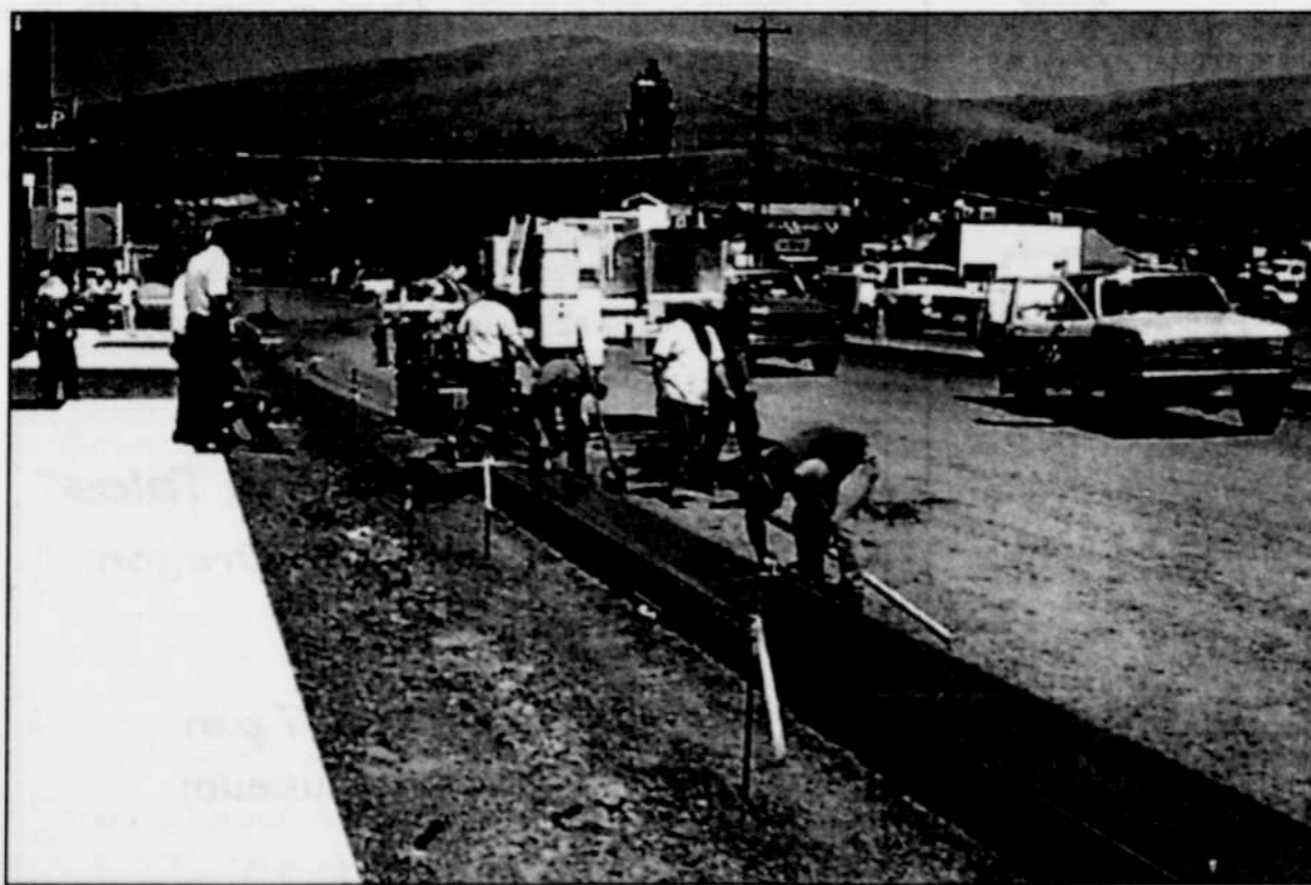
Curbs nearly completed on west side of Main Street
