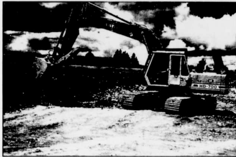
Backhoe begins work at new Heppner subdivision
