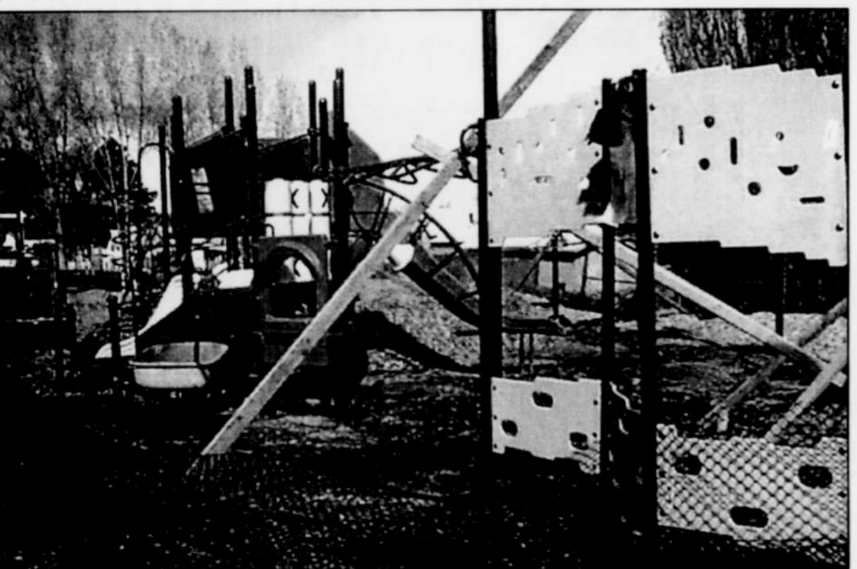
Almost finished-just waiting for the cement to set.
