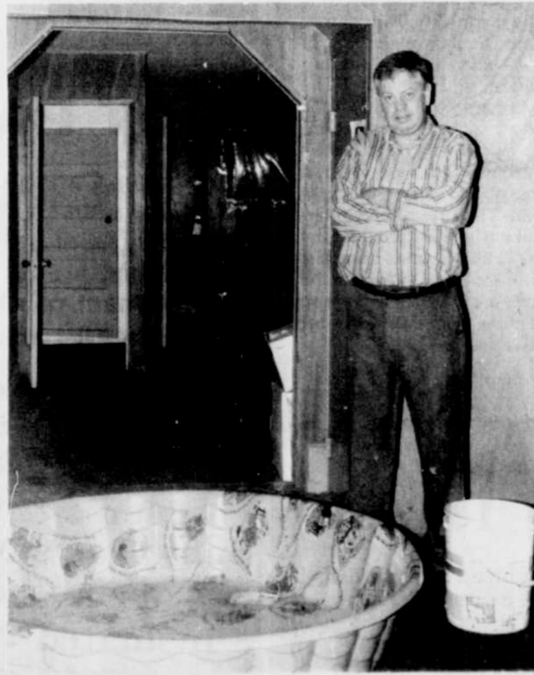
Bob Ployhar uses wading pool to catch leaks
