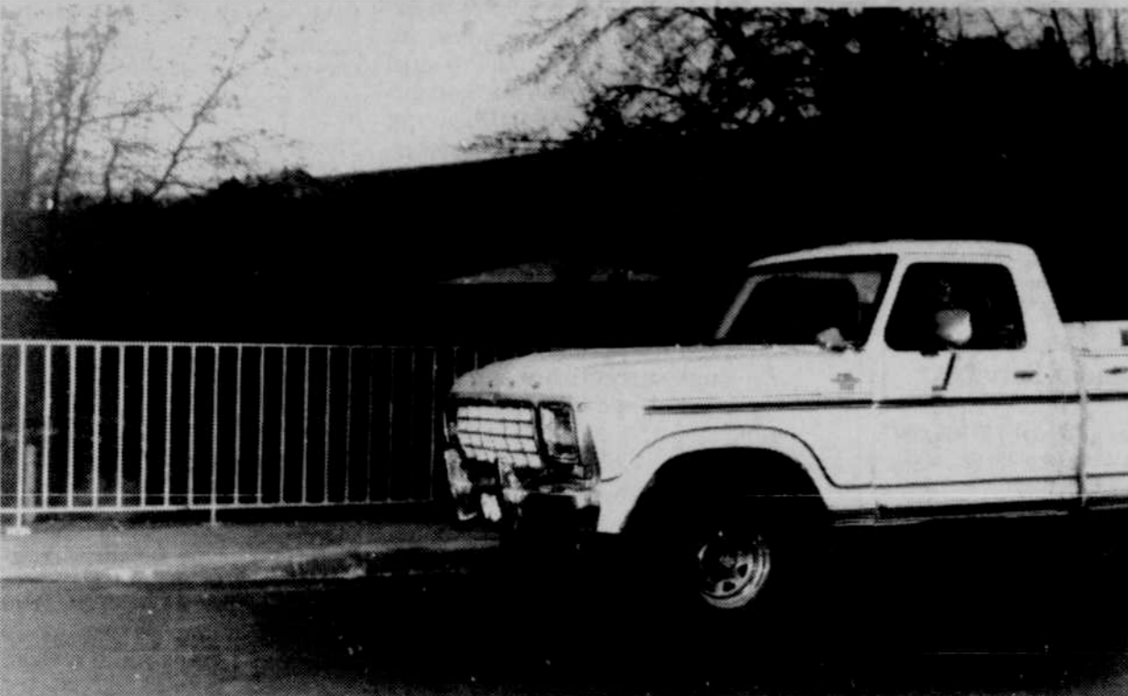
Pat Sweeney drives across newly completed Court St. bridge
