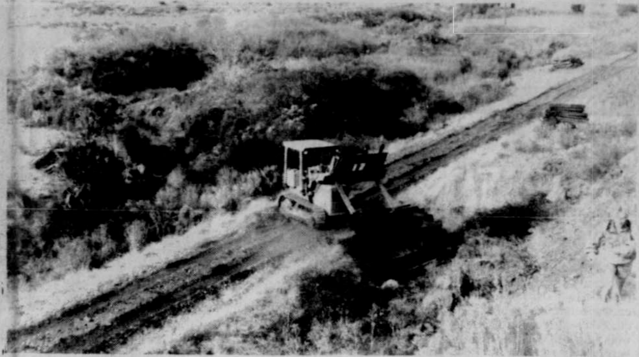
Korey Richins with A&K Railroad Materials, Inc., picks up railroad ties with a forklift.
