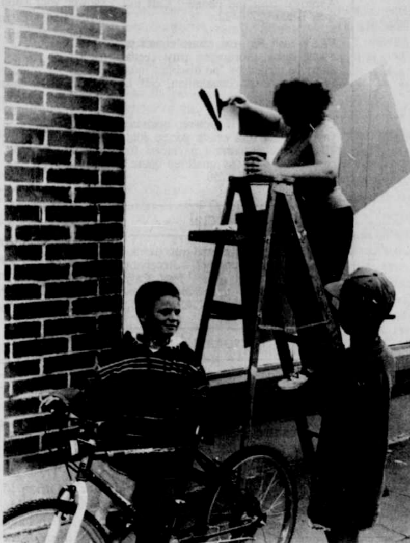
Casey Childers (left) and Adam McCabe watch Tonya Heideman paint the lone Cycle Oregon logo "Yikes Bikes" on a downtown building.
